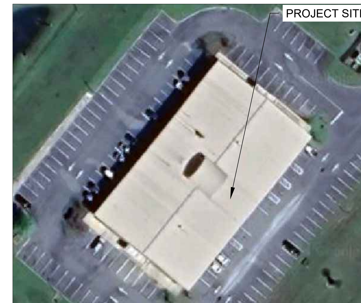
1 BUILDING PHOTO SCALE: NTS
